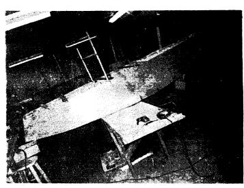
First newsletter pictures are of the KR-3 fuselage under construction. Note the wing rib at mid fuselage. The clamped on crossbar is 16" above the top longeron, that is the height of the bubble canopy. Wing spars have been installed since pictures were taken.
